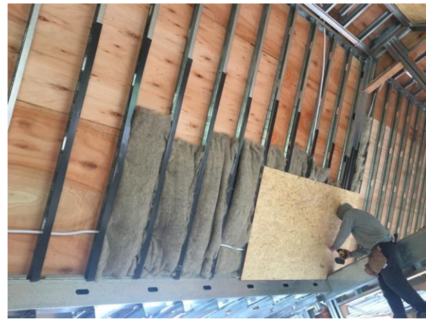
Figure 6: sheep wool insulation blankets installed in La Escocesa. a house in the Province of Buenos Aires.
