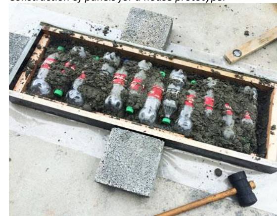
Figure 2: Construction of panels for a house prototype.
