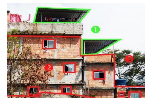
Figure 3: Multi-story residential building cluster in the Favela of Paraisópolis, Sao Paulo, showing a sequence of shaded roof tops, bare brick walls and standardized aluminum windows.
