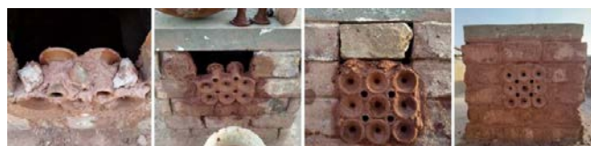
Figure 3: The construction process of the eco-cooler during the proof-of-concept test cells using 8 and 16 funnels.
